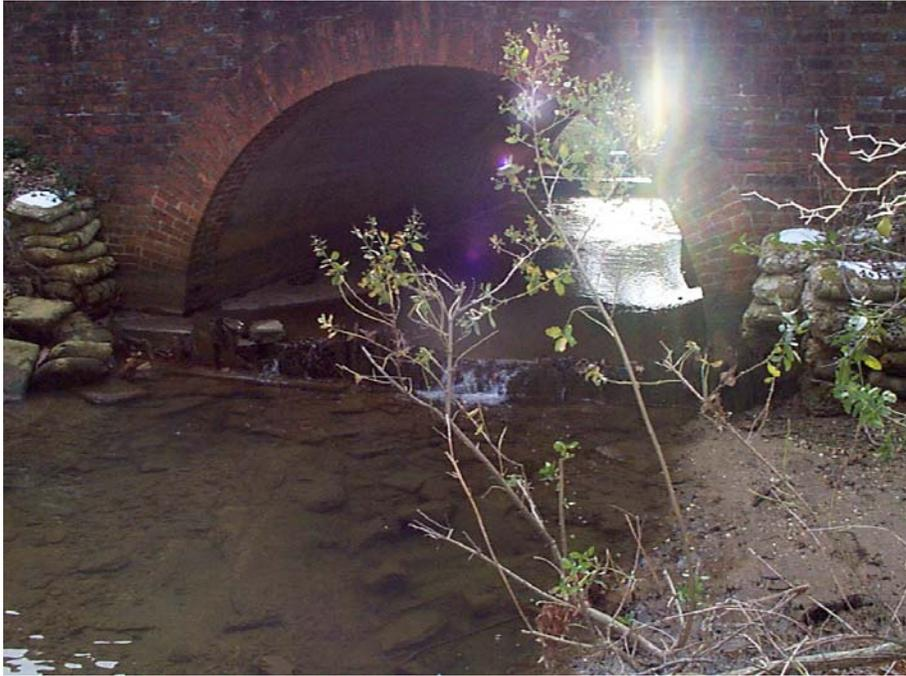
Figure 3. Bridge over Wormley Creek with Wormley Pond in background. Irish ramp was set under the bridge at the base of the dam near the right wall.
