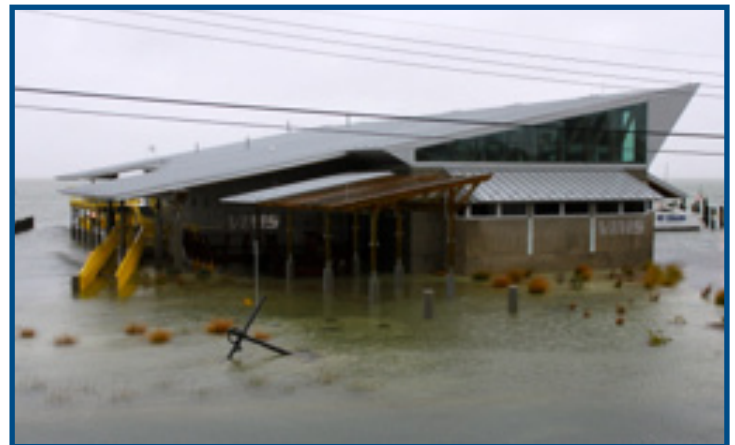
The new seawater facility at VIMS’ Eastern Shore Lab in Wachapreague stayed dry as designed during minor coastal flooding associated with Hurricane Sandy.
