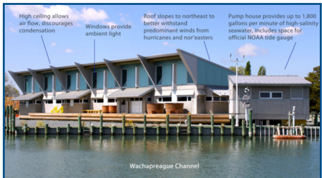
Form Follows Function: The new seawater lab incorporates numerous design functions that enhance its use as a research and teaching facility.
