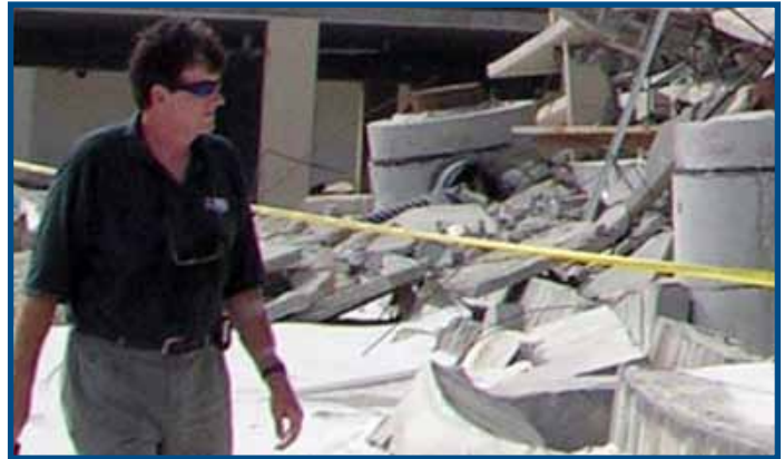
Storm Impact: Sallenger surveys the aftermath of Hurricane Ivan in 2004 on the Panhandle of Florida near Pensacola. Standing adjacent to a high rise condo whose lower floors had been blown through by waves and surge. Photo courtesy of USGS
