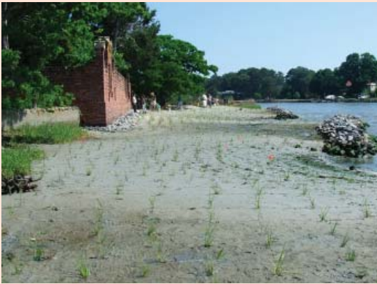
Medium energy eroding marsh before (above) and after living shoreline treatment (below). Photos of Hermitage Site by Walt Priest
