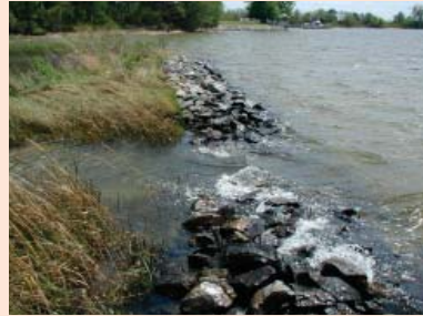
Offset (above) and straight gaps (below) maintain connections to shoreline habitat and open water.
