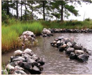
Offset (above) and straight gaps (below) maintain connections to shoreline habitat and open water.
