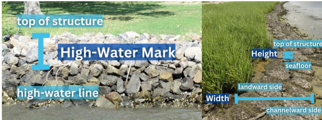
Fig 18. Structure measures on a rock sill and oyster reef structure.
