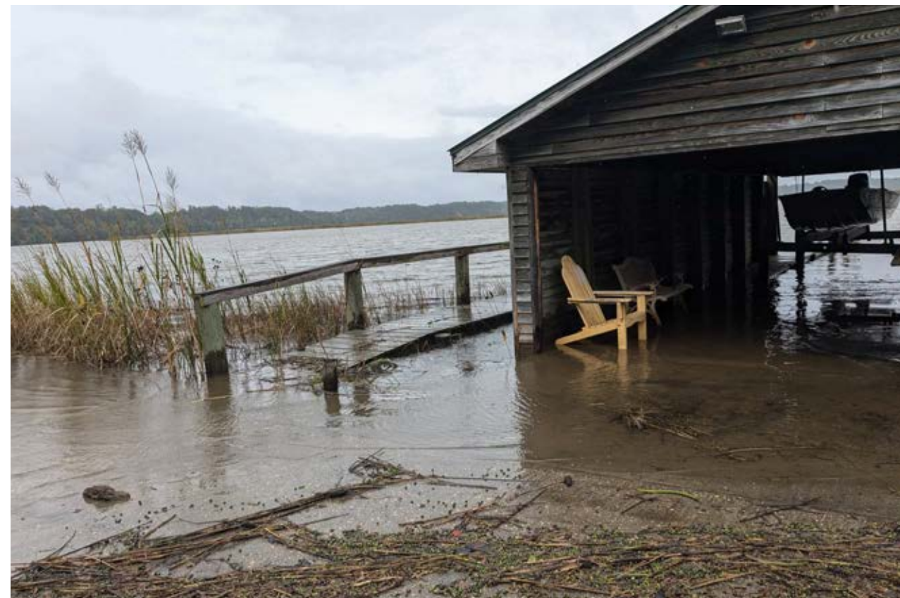
Flooding of a shoreline residence in the York Watershed System. Credit: CBNERR-VA.
