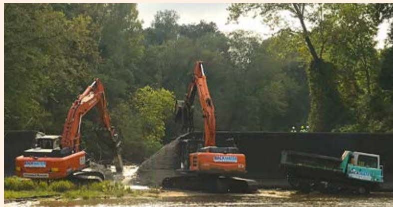
Heavy machinery works to demolish and remove the 1916 Ashland Mill Dam making way for migratory and resident fish species. Credit: Alan Weaver.
