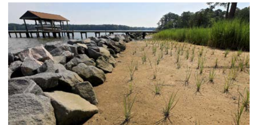
Completion of a living shoreline installation in York Watershed System tidewaters. Credit: Consociate Media.
