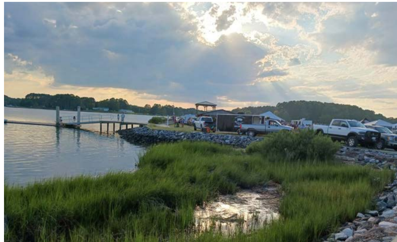
A hybrid shoreline at Williams Wharf Landing in Mathews County, VA. Credit: D. Frantz
