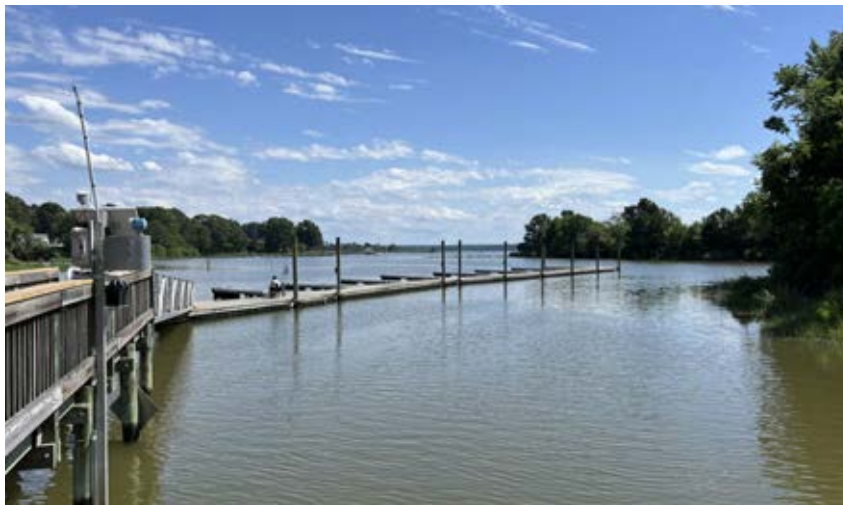
Boat slips at Machicomoco State Park. Credit: CBNERR-VA.
