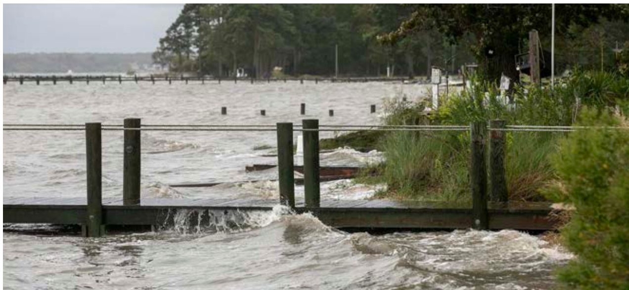
Storm surge batters shorelines in York Watershed System Tidewaters. Credit: Consociate Media.
