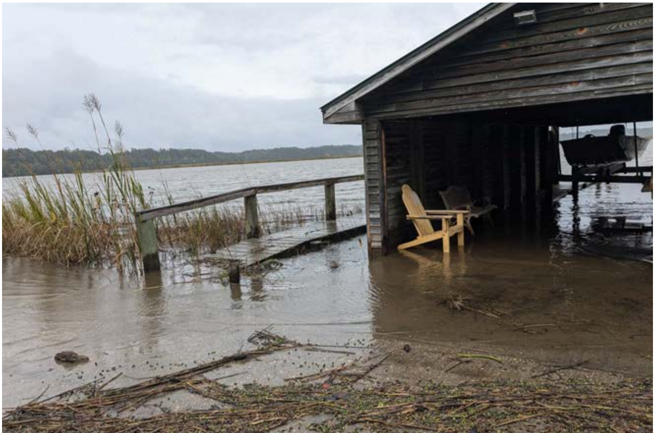
Flooding of a shoreline residence in the York Watershed System. Credit: CBNERR-VA.
