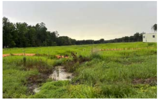
Sediment-filled stream at a future construction site within the York Watershed System. Credit: CBNERR-VA.
