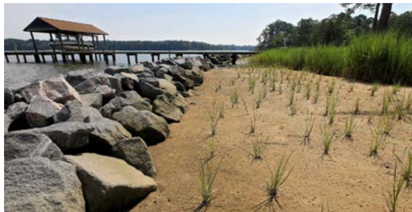
Completion of a living shoreline installation in York Watershed System tidewaters. Credit: Consociate Media.
