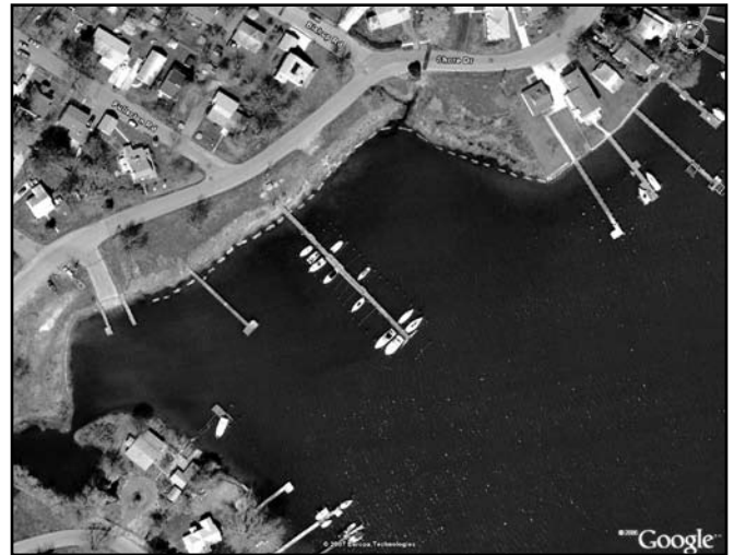
Figure 1. Placement of 33 segmented stone sills to create a living shoreline along 750 linear feet of shoreline in Glebe Bay, South River, Maryland
