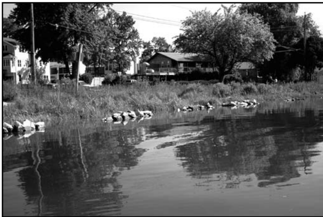
Figure 2. 12-foot long sills with 6-foot windows at the living shoreline site in Glebe Bay, South River, Maryland.
