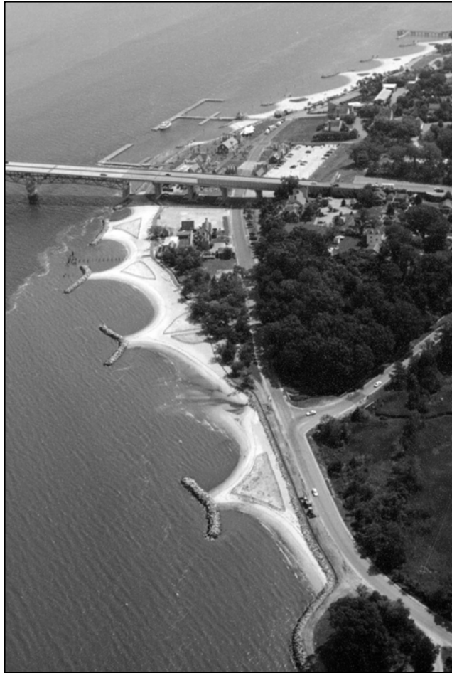
An aerial view of the Yorktown waterfront shows the breakwaters that protect the new Riverwalk development.
