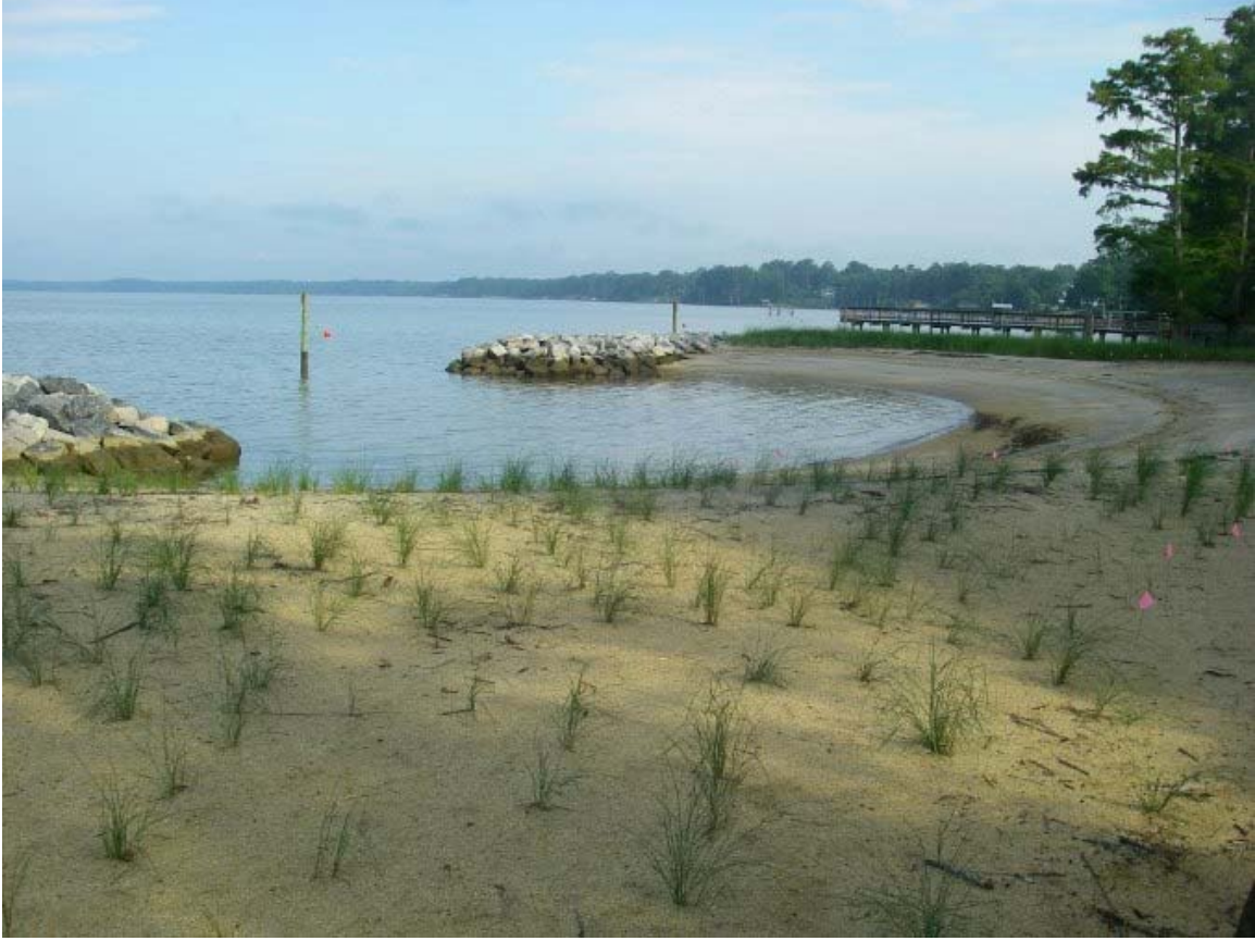
Figure 3. New breakwater constructed at J36 on the James River overlaying the historic sampling location. For 2011, the seine location was moved approximately 100m upstream (just beyond the dock in the right background).
