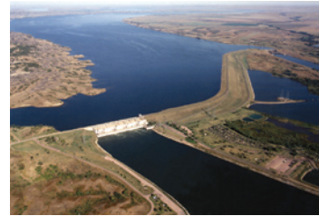
Fort Thompson Big Bend Dam, USACE Digital Visual Library
