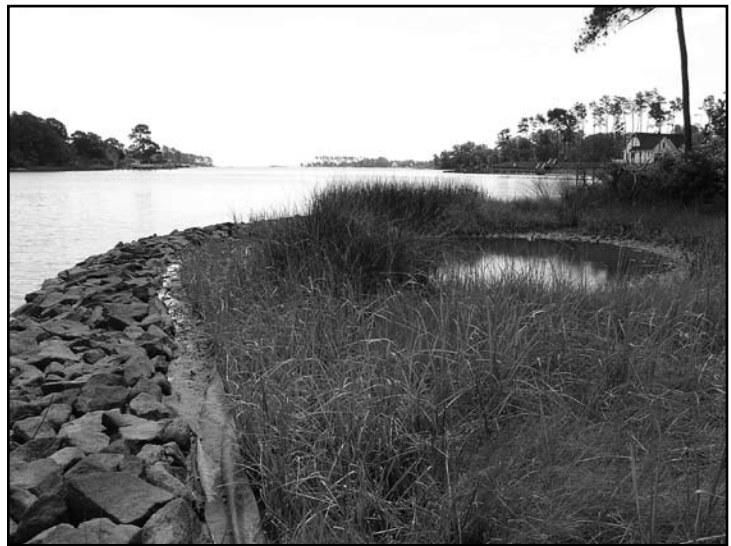
Figure 1. “Marsh toe revetments” are placed next to the edge of an eroding tidal marsh.
