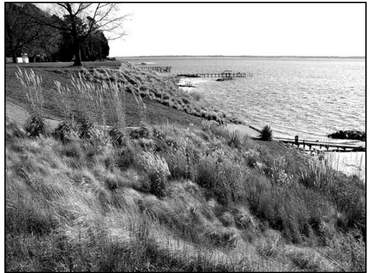
Figure 4. A previously vertical, eroding bluff was graded and planted with native and ornamental grasses.
